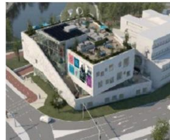
Joint Research Center Zeeland
