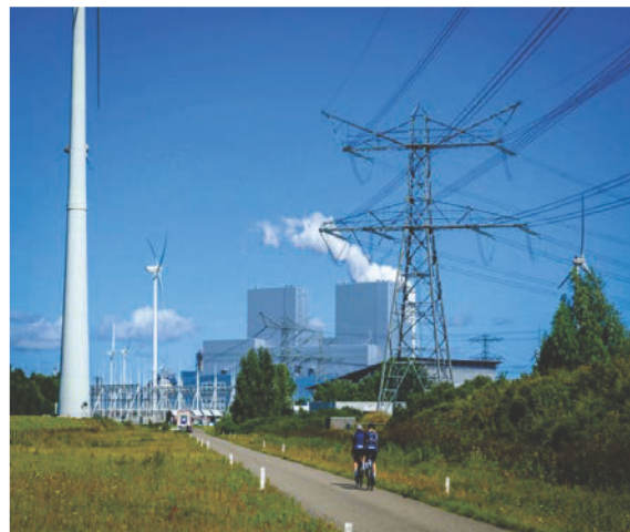
Windpark RWE, Eemshaven
