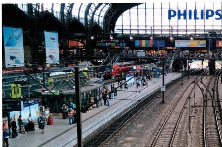
Hamburg Hbf with 2 trains of different service contracts on platform 6
